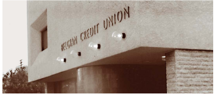
Belgian Credit Union's new building shortly after it opened in 1975
